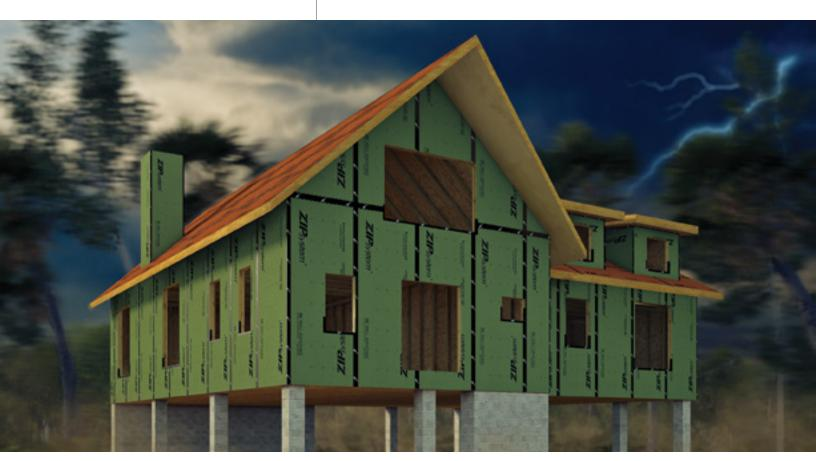
11 The built-in, water-resistive, vapor-permeable barrier is ideal for waterproofing, which is of the utmost importance for any construction project.
