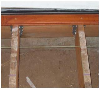
2-5 rows of TigerDeck® deck boards (or the entire deck) can then be laid out on the joists with one clip on each joist. Do not screw the clips down as you go. Push everything in place with hand pressure and set up Bow Wrench(s) in preparation for squeezing a 2-5 row section tight. Natural bow should be placed with the belly out.
