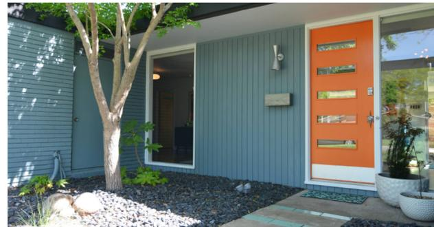
Plywood siding is 4x8 panels with machined paneling/grooves that is approved for exterior siding. It is easy to install, low cost, and very attractive. There are two grades - Premium & Deco. Our Deco grade will have imperfections and patches that are repaired with glue and adhesive and is intended to be painted. Premium siding can be stained or painted and will have minimal patches and repairs and a very high quality finish.
