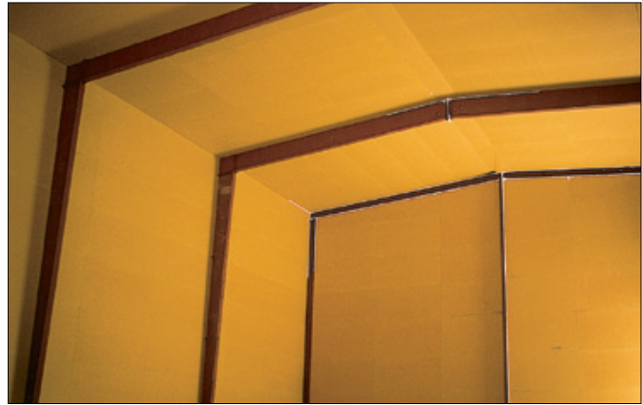
MDO panels are applied to the interior of a cold storage building.
