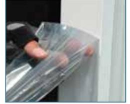
When installing other products such as HardiePlank® Lap Siding and HardiePanel® Vertical Siding with ColorPlus® Technology, leave the protective laminate sheet on the board during cutting and installation. Once the product is installed the laminate sheet should be removed.
