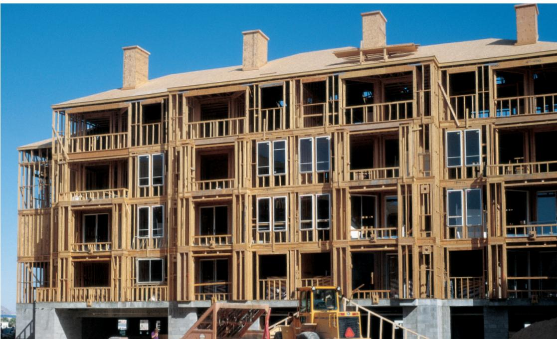
High-performance visually- and mechanically-graded products are well suited for multistory and pre-engineered applications.
