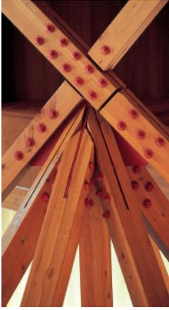
Exposed, load-bearing glulam beams bring handsome elegance and a sense of warmth to engineered heavy-timber framing.
