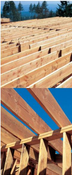
Douglas Fir and Western Larch dimension products are the ideal framing material. The combination of high MOE and  $F_b$  design values provides a high degree of stiffness which is particularly desirable in floor systems. The higher grades in this exceptionally strong species group perform competitively with many engineered products and are more economical.
