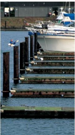
Pressure-treated Douglas Fir pilings and boardwalks were used for this salt-water marina in Newport, OR.
