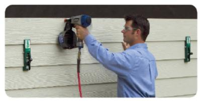
A Nail siding per manufacturer's recommendations. Remove both gauges and repeat steps 1 though 4 as you work upward to top of wall.
