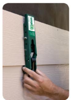
At approximately one-third of your siding's overall length from either end, place the Gecko's blade under bottom edge of siding and slide upward.
