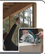
Tip: It is easier to cut the column wrap to length prior to removing all the shrink wrap
