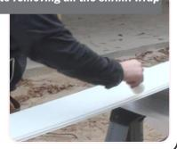
Place the three sided section of the wrap around the column. Make certain that the wrap is as plumb as possible (shims may be necessary). Secure the wrap to the column placing a weather resistant screw at
