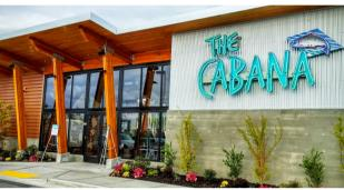
**Treated Glulam Beams** are pressure treated with a Hi-Clear II, a clear industrial wood preservative. It leaves a light honey color finish that is virtually undetectable to the naked eye. It is intended for above-ground exterior applications and is most common for raised deck beams.
