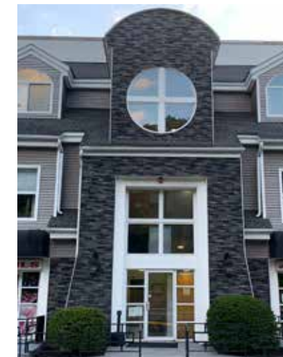
Stacked Stone - Lewiston Crest
